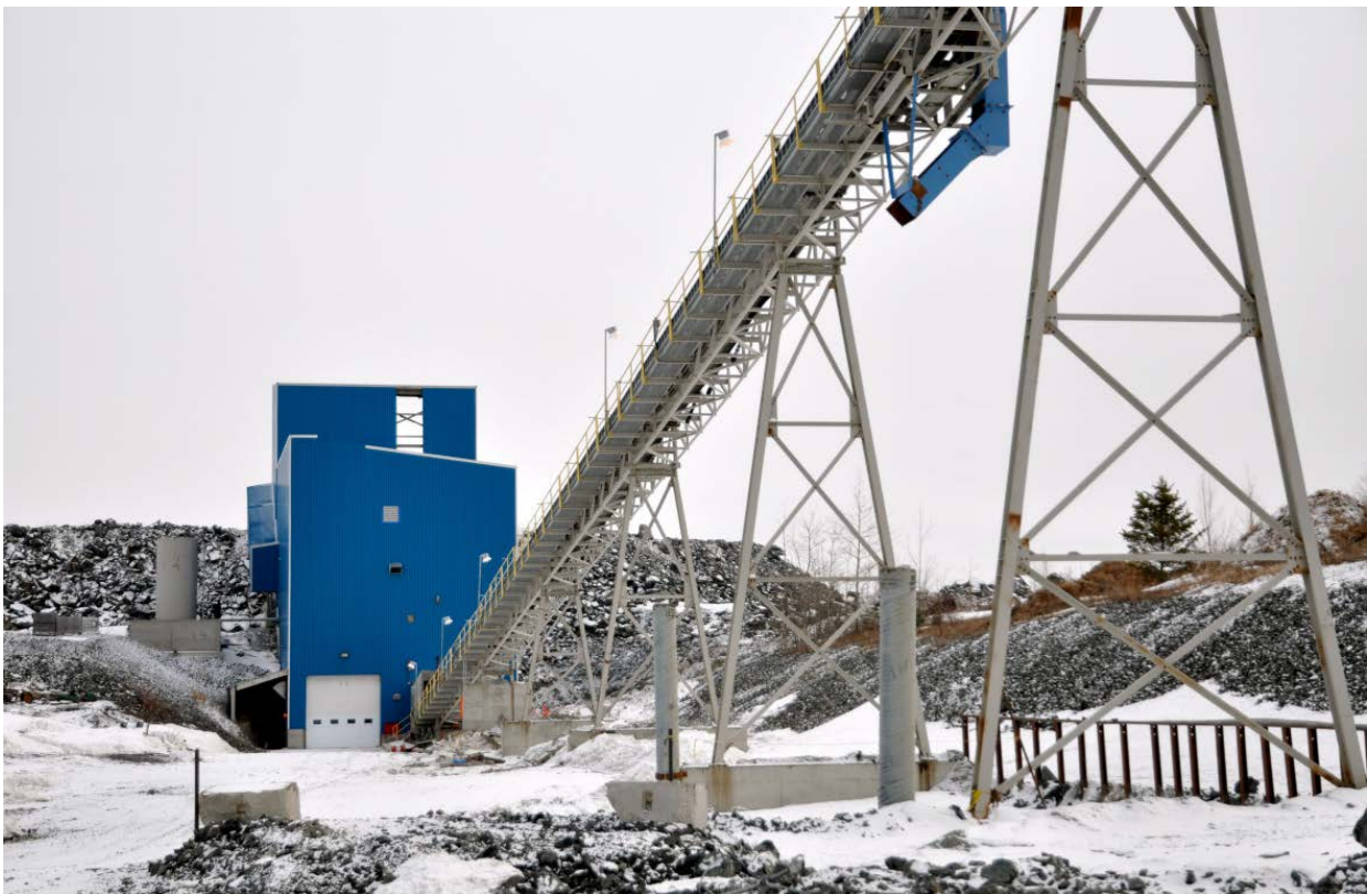
Crusher and conveyor
