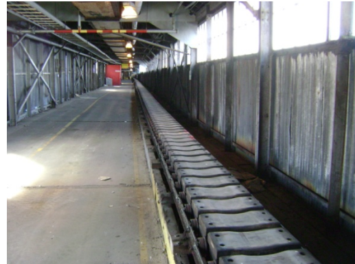
1929 Wood Slat Conveyor
