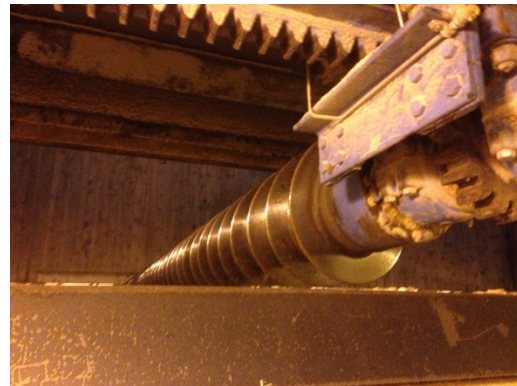
Screw Conveyor in A Frame Building
