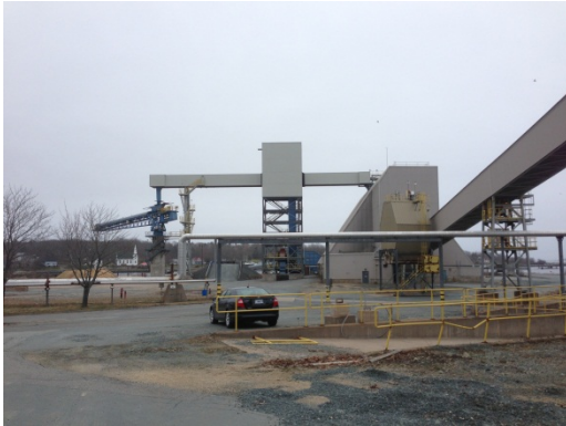
Conveyors to A-Frame Building
