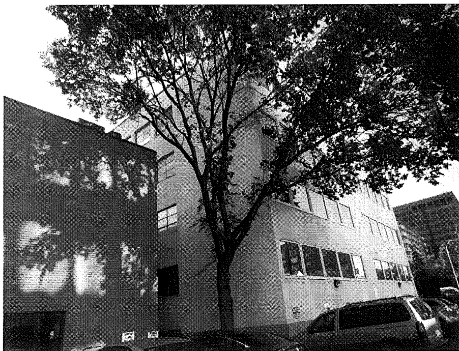
View of the Commonwealth Building from the Northwest
