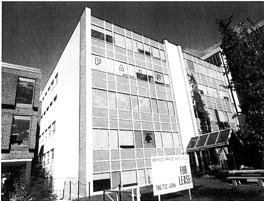
View of the Commonwealth Building from the Southeast
