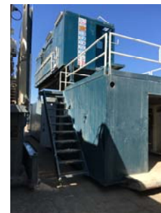
2.6 Water Tank and Dog house
