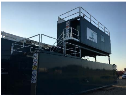
3.6 Water Tank and Doghouse
