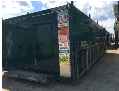
1.5 Mud Pump Building
