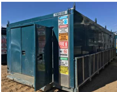
2.5 Mud Pump Building
