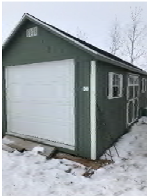
Storage Shed with Rolling Door
