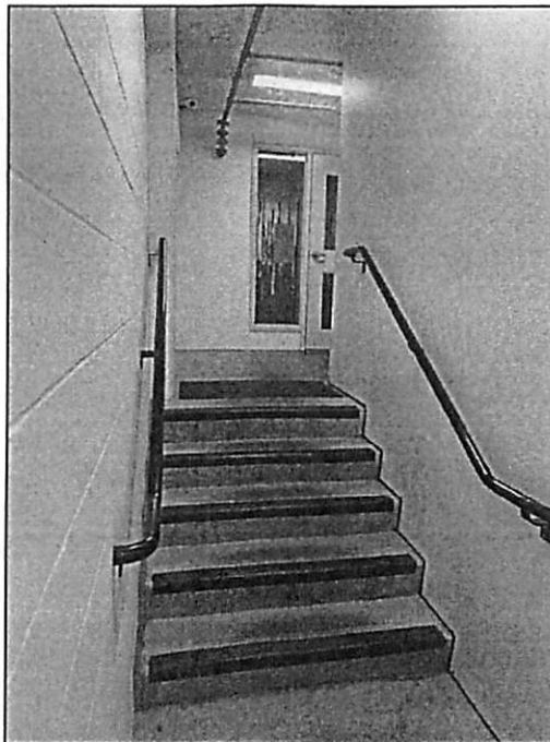
View of access from parkade to the Versante Hotel
