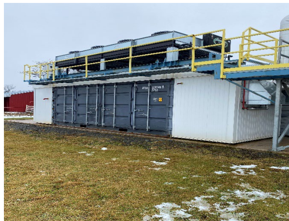
20ft Container with Frick Rotary Screw Compressor System (Wired and Installed) Package
