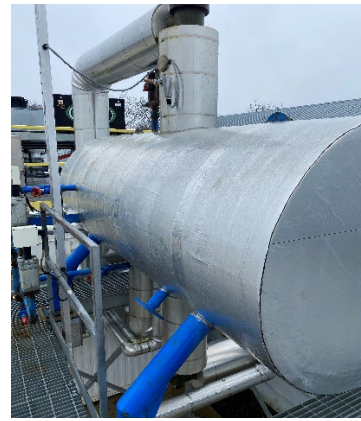
Low Pressure Receiver Tank Tunnel Freezer Refrigeration
