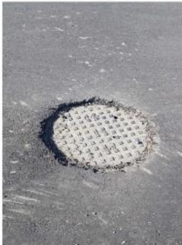
Photo 3 – Manhole Requiring Adjusting
