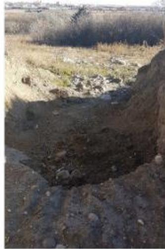
Photo 6 – Backfill Erosion Trench
