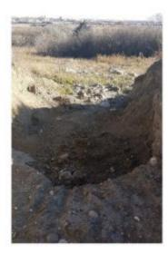
Photo 6 - Backfill Erosion Trench
