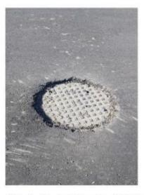
Photo 3 - Manhole Requiring Adjusting
