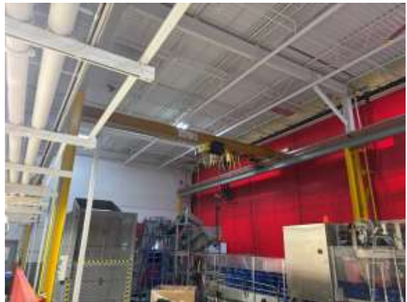
Subject Improvements – Warehouse/Manufacturing Area
