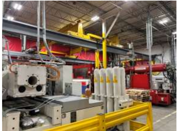
Subject Improvements – Warehouse/Manufacturing Area
