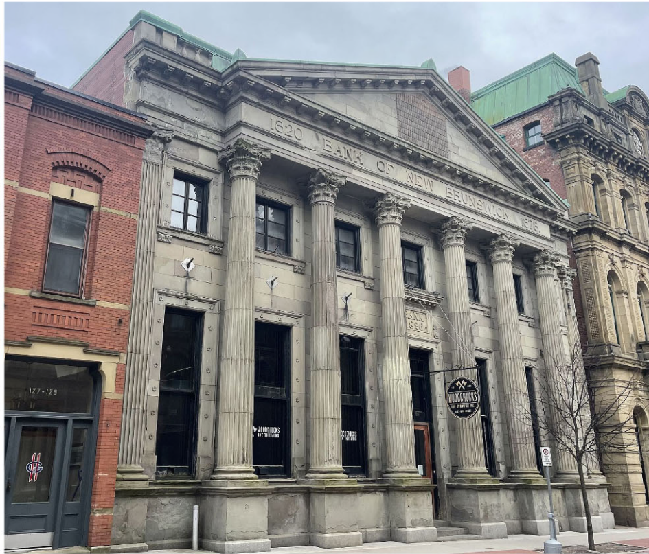
Subject from southeast
