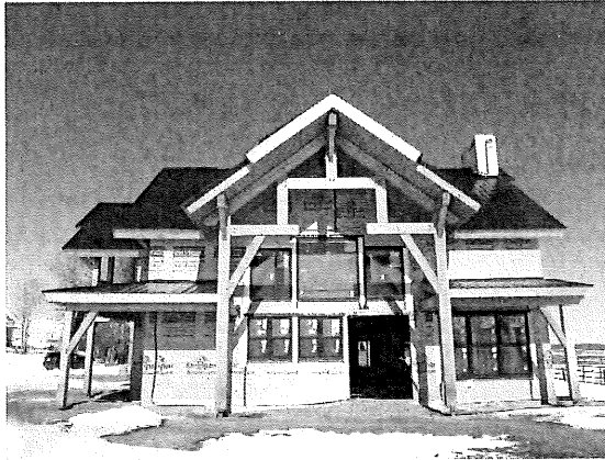
View of South Façade of House
