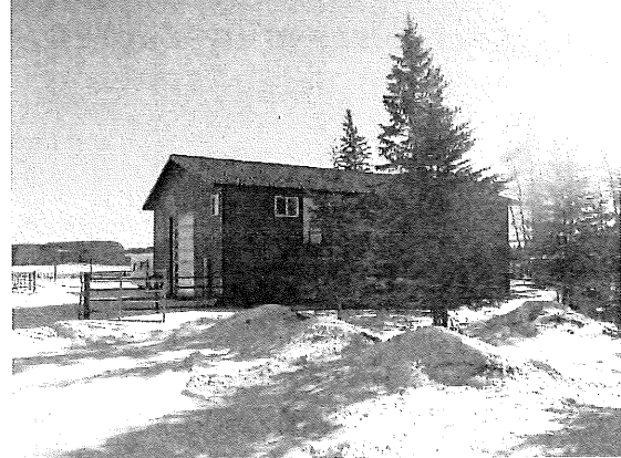
View of New Shop Building
