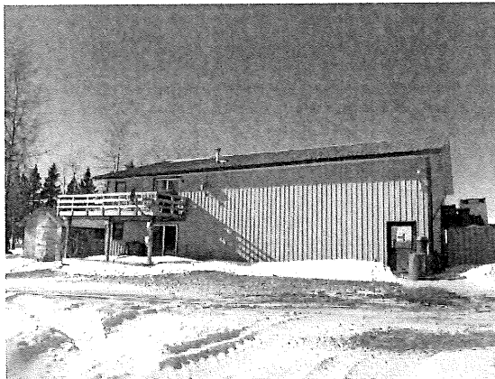
View of 2006 Shop Building
