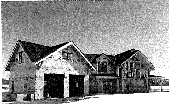
Partially Completed Single Family House
