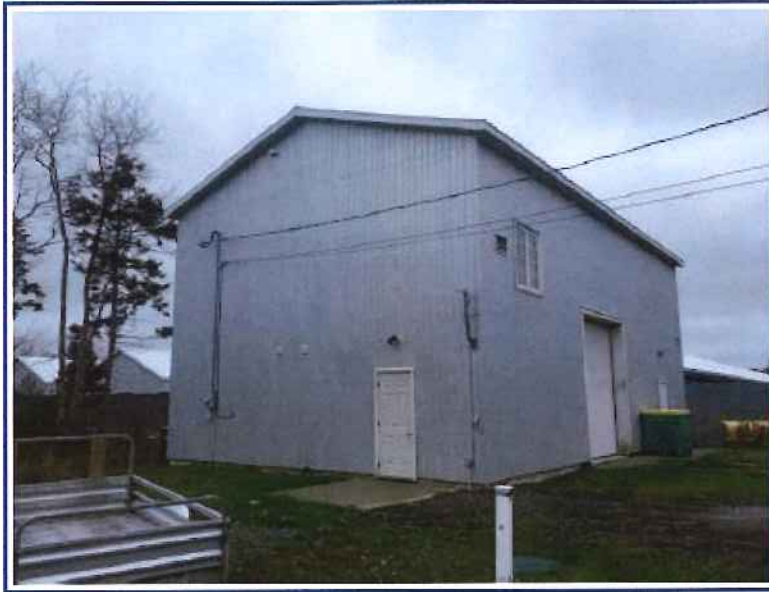
Front view of office/shop building
