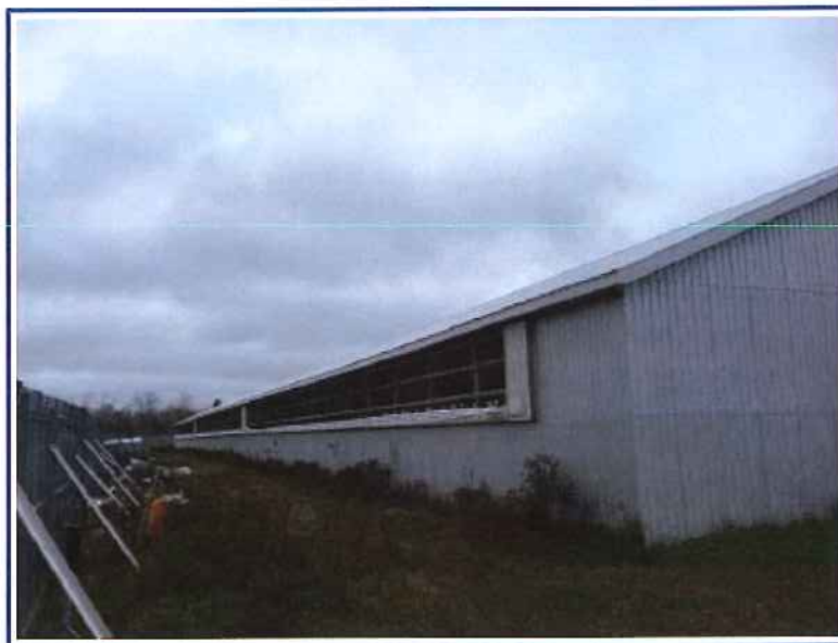
View along side wall of mink barn
