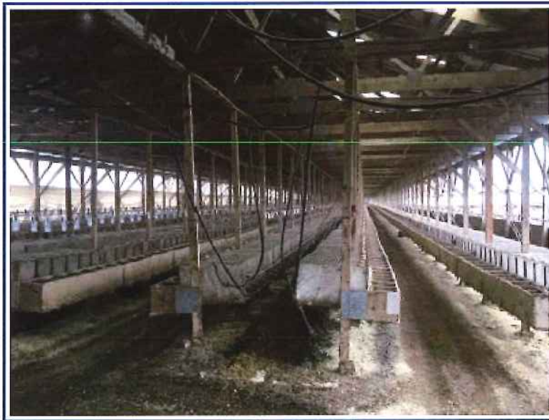
Interior view of four isle mink barn
