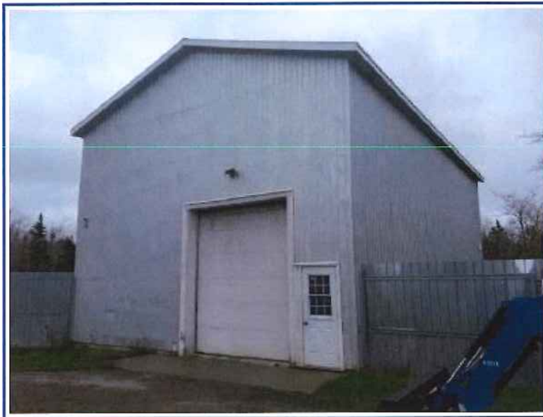
Rear view of office/shop building
