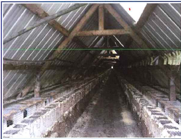
Interior view of single isle mink barn
