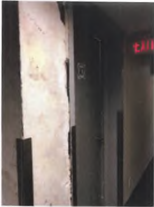
345 – 7th floor water damaged wall between elevator and stairwell door
