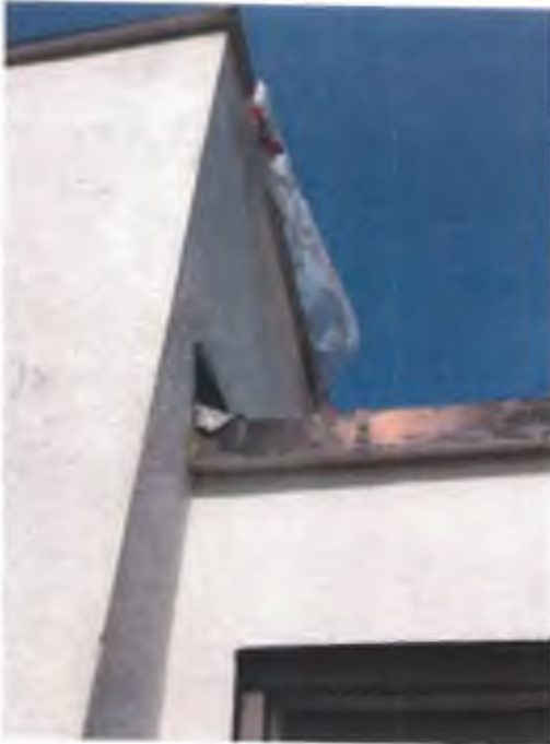
345 - mechanical room roof
