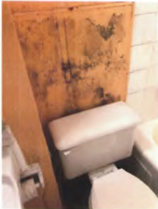
345 – apartment 709, water damaged bathroom walls, black mold is present
