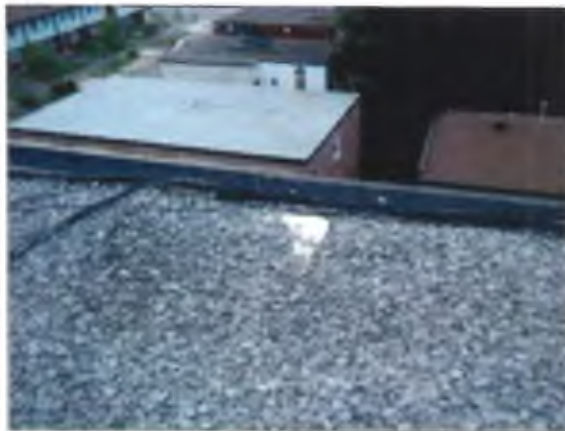
View of exposed insulation within the original portion IRMA system.
