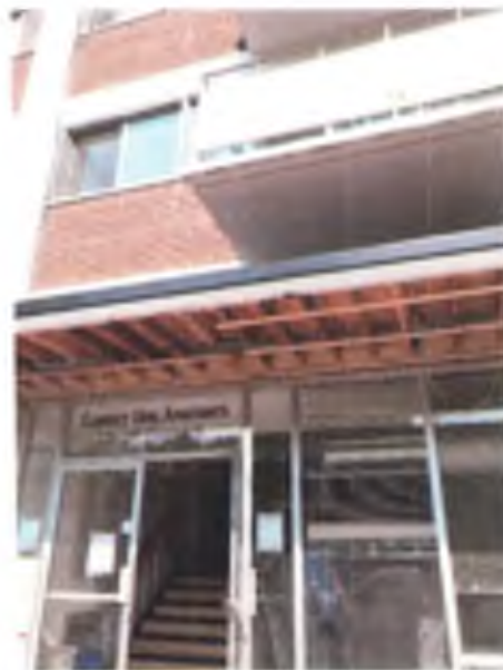
345 – front entrance canopy repairs
