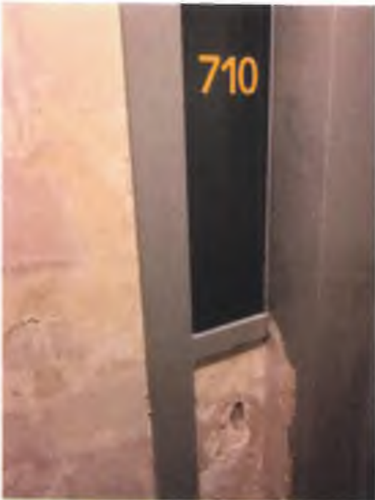
345 – water damaged hallway wall beside apartment 710
