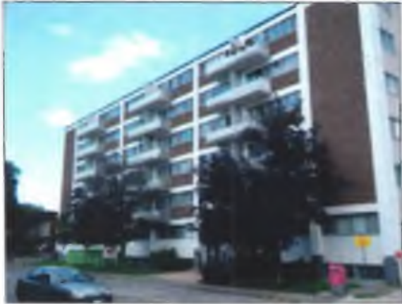
General view of the south elevation of the Site Building.
