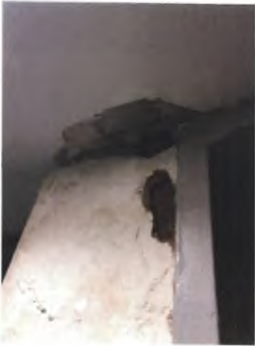
345 – 7th floor water damaged wall between elevator and stairwell door
