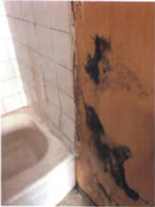
345 – apartment 709, water damaged bathroom walls, black mold is present
