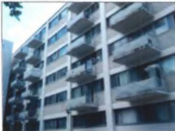
General view of the north elevation of the original portion of the Site Building.
