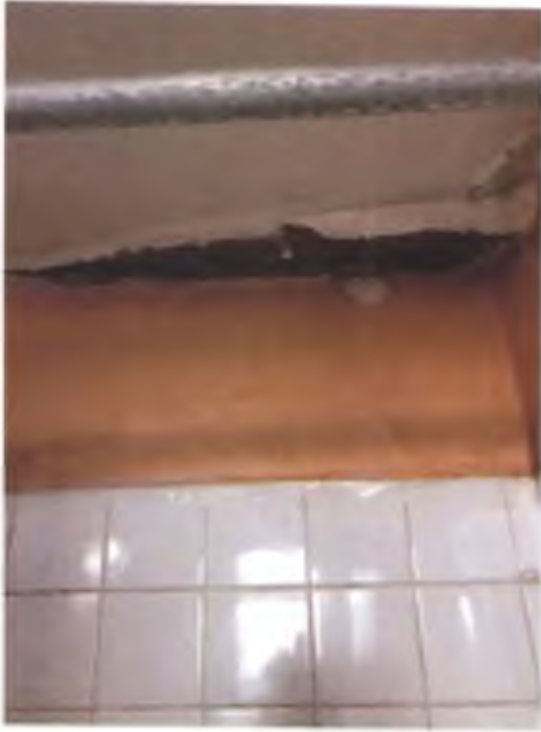
345 – apartment 709, water damaged bathroom ceiling
