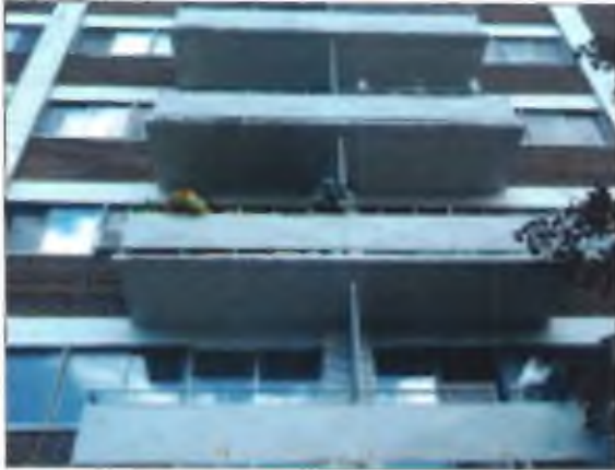
View of the typical balconies of the Site Building.
