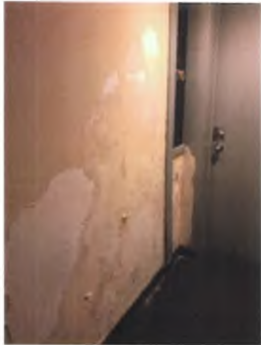
345 – 7th floor water damaged wall between elevator and stairwell door
