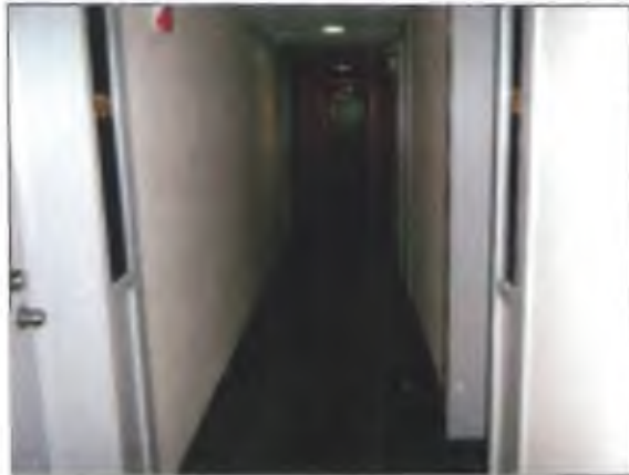
View of the finishes within a typical corridor.
