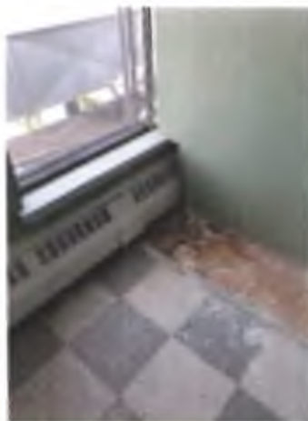
345 – patio door, water damaged drywall 345 – patio door, water stains on parquet flooring
