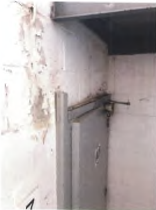
345 – stairwell below roof access door
